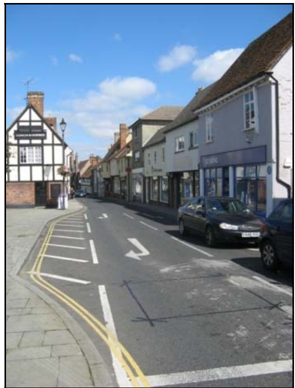
This 2 lane section to be moved to the left to include the hatched area, with the kerb approaching the stop line realigned.
