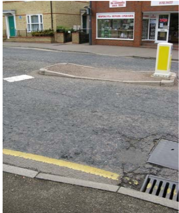
This photo shows the current unofficial pedestrian crossing on Baldock Street, hard up against the mini roundabout outside Morrisons.
