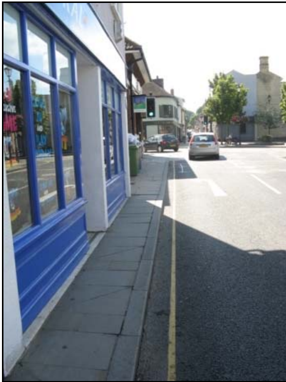
The narrowest section of footpath on Kneesworth Street approaching The Cross, to be widened to a minimum of 2 meters
