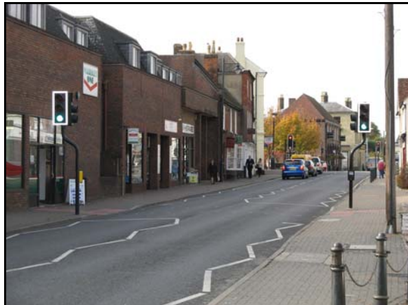
This photo shows the existing site of the pedestrian crossing on Melbourn Street, in relation to the nearby Cross signals
