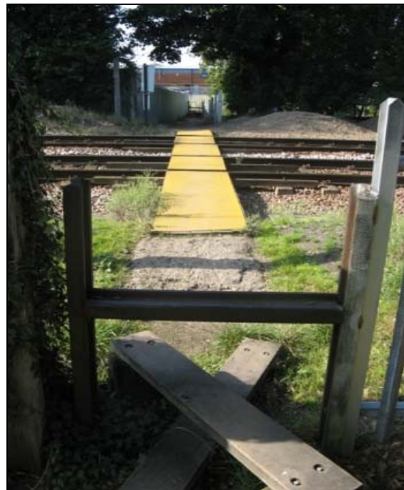
West Rail Pedestrian Crossing access
